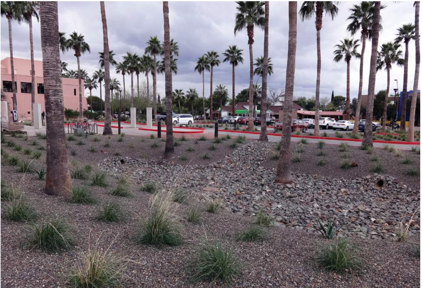
Figure 7.4 Bioswale on Arizona State University Campus to Capture Rainwater Runoff from a Parking Lot
