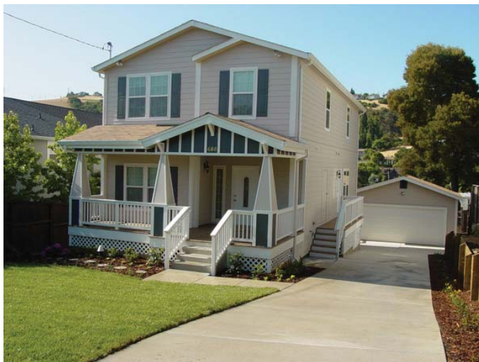
Figure 8.2: Modular home constructed and transported in four modules, enhanced on-site with porch and detached garage
