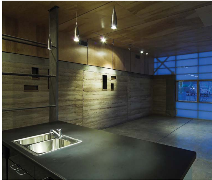
Figure 15.3: Rammed earth wall of an affordable housing unit
