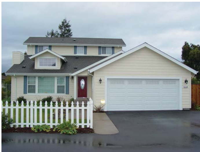
Figure 8.1: Two-story manufactured home consisting of three factory-built sections, completed with the on-site construction of a garage
