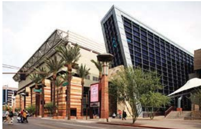
FIGURE 6 | The Phoenix Convention Center incorporates energy-efficiency design in order to achieve 20% energy savings from lighting and HVAC controls technologies and water savings from low-flow urinals, dual-flush water closets, and low-flow lavatories (saving 1.9 million gallons per day). Building and construction recycling efforts diverted over 84% (3,100 tons) of material away from the landfill. 18
