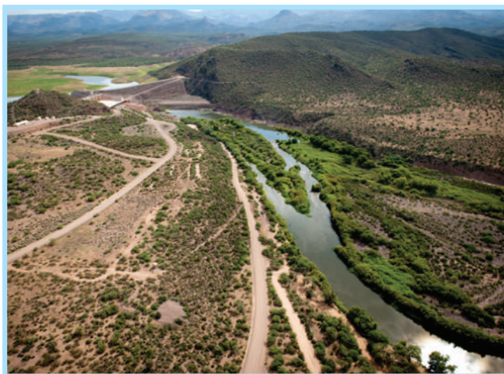
Horseshoe Dam, an earth-fill structure 194 feet high on the Salt River in Arizona. Source: U.S. Bureau of Reclamation, Andrew Pernick.
